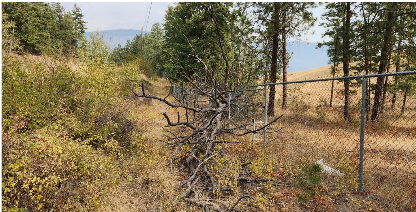
Photo 1: Damaged perimeter fencing along western property boundary due to fallen tree, facing northeast. 11 Sept 2023.
